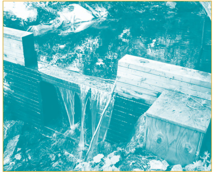
Figure 12. Intake for a 2-kW micro-hydropower system (photo courtesy of Homestead Hydro Systems)
