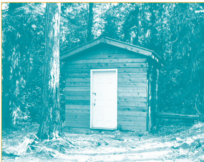
Figure 16. Powerhouse for an 8-kW system (photo courtesy of Thompson and Howe Energy Systems Inc.)
