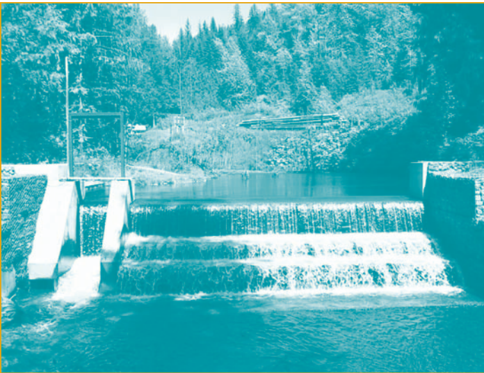
Figure 10. Intake of micro-hydropower system in Seaton Creek, British Columbia (photo courtesy of Homestead Hydro Systems)
