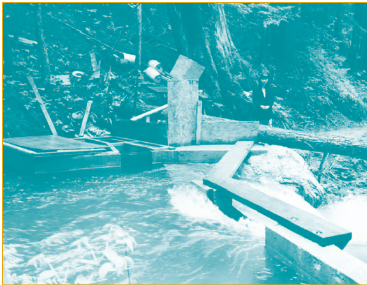
Figure 11. An intake weir for a 7-kW system (photo courtesy of Thompson and Howe Energy Systems Inc.)
